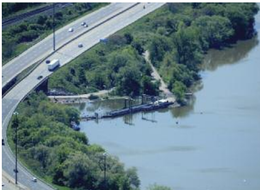
The eastern end of Cootes Paradise Marsh terminates at the Cootes Paradise Fishway, the black structure which controls the passage of fish to and from the marsh.
