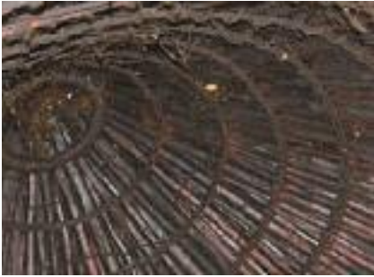
A hut roof constructed from local timber (Alex Hudson)
